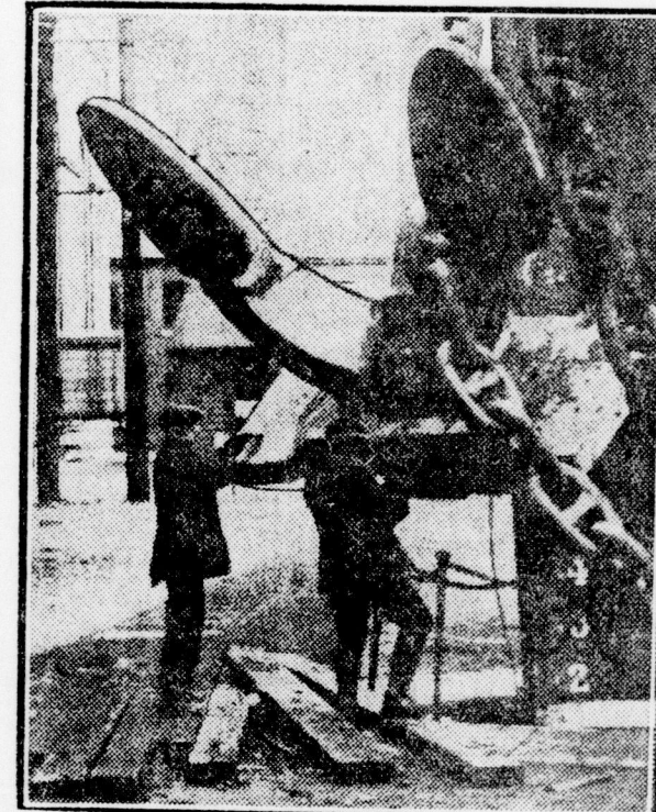
Here's where the old "mud hook" gets its manicuring. One of the huge fifteen-ton anchors of an ocean liner is seen being scraped during the steamer's annual overhaul in dry-dock at Southampton.
