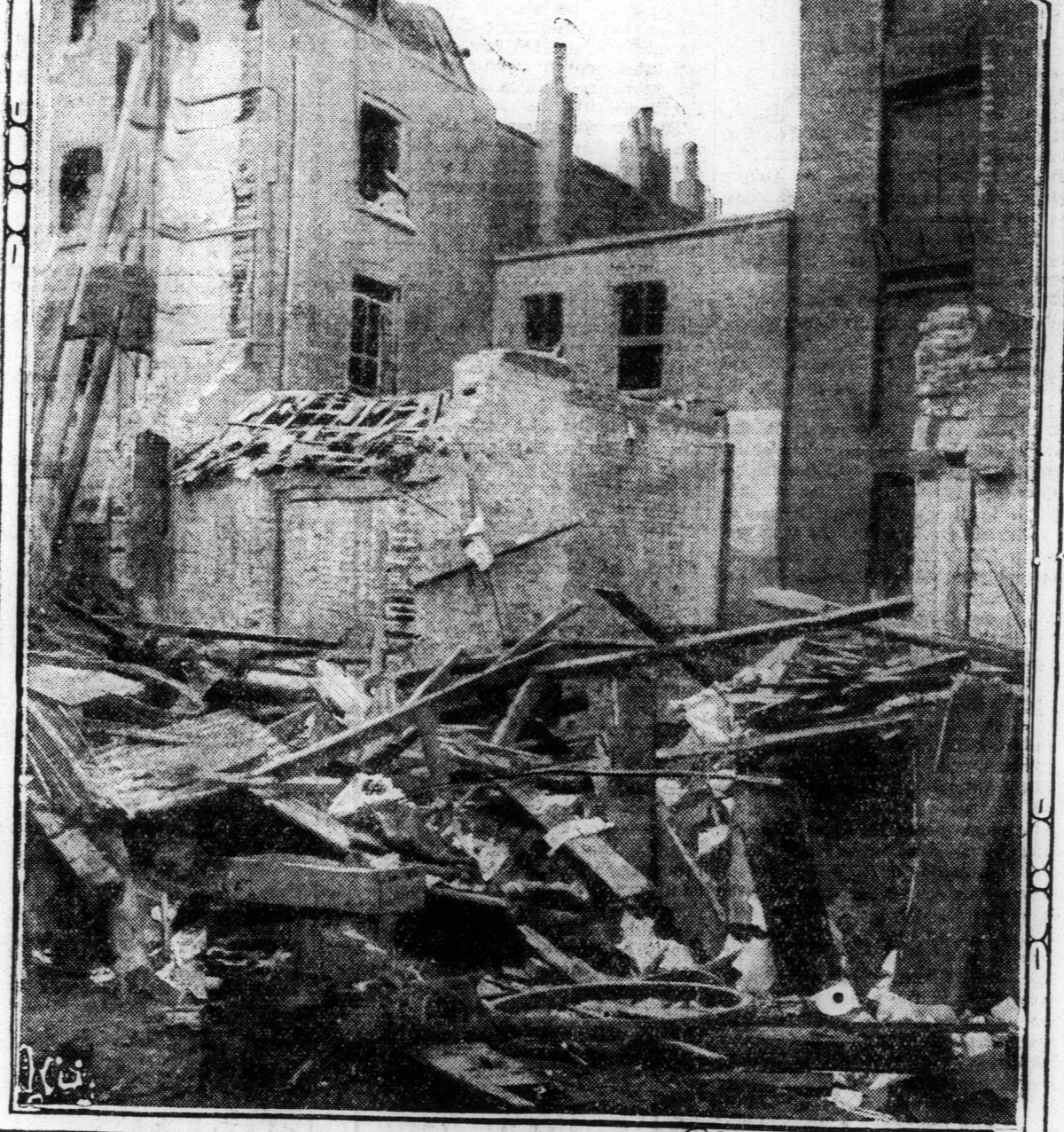
CLOSER VIEW OF WRECKED WORKING-CLASS PROPERTY PHOTOS BY WALSHMAN
