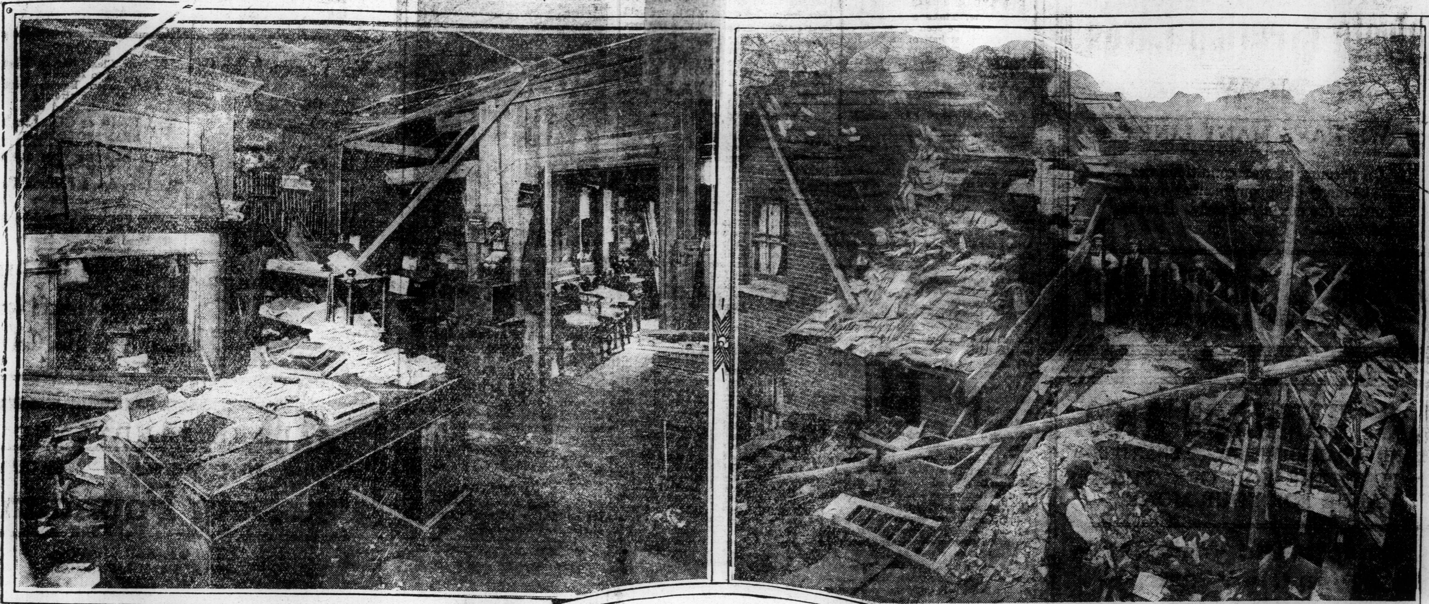
INTERIOR OF A ROOM USED FOR BUSINESS PURPOSES THE DAMAGE SHOWN WAS CAUSED BY THE EXPLOSION OF THE BOMB OUTSIDE
