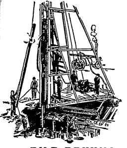
on land or water by Steam Pile Drivers or Drop Hammers.
