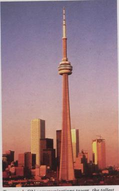
Toronto's CN communications tower, the tallest free-standing structure in the world, houses microwave antennas and equipment for radio and television broadcasting.
