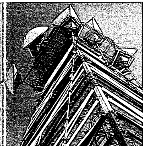
Digital Microwave . . . One of the towers in TELECOM CANADA's dual transcontinental chain of microwave radio routes. A substantial portion of this network operates using digital transmission techniques.
