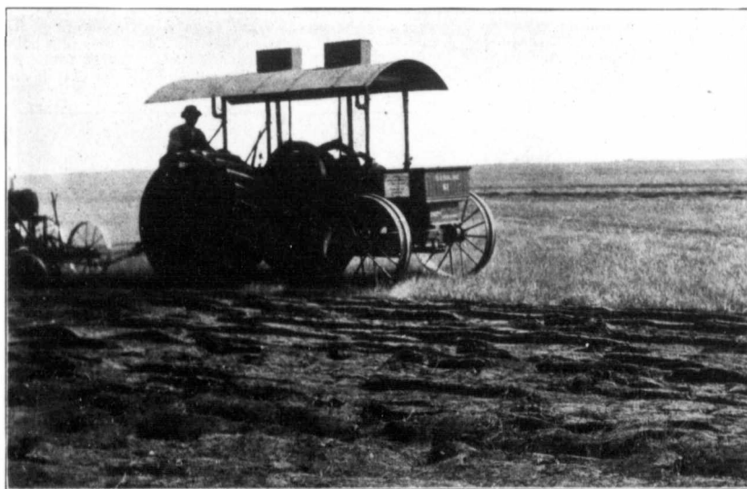
Goold Shapley & Muir 20 h.p. Gas Tractor in the contest. This engine pulled 3, 2 bottom 14 in. Imperial Gangs. The photographer miscalculated and mapped only the engine at work
