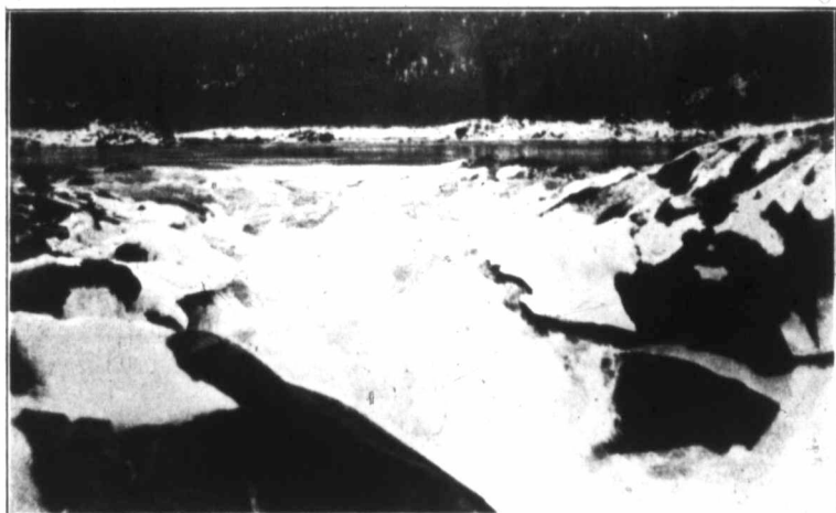
Site of Power Plant.
