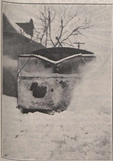
Rear end of rotary snow plough, Levis County Ry. showing cutting blades and fan paddles, which run at 1,200
