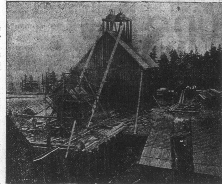
SHAFT HOUSE, TYE MINE.
