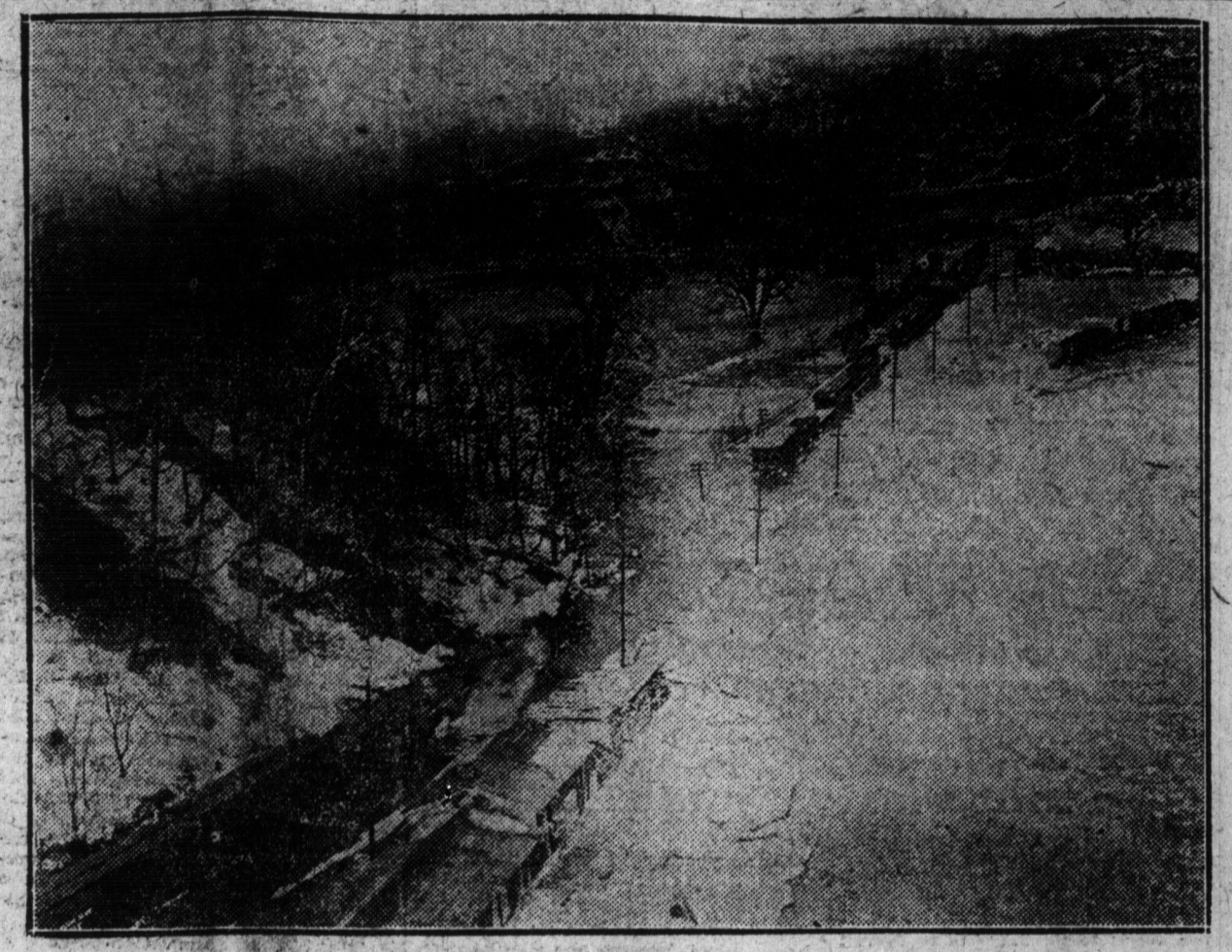
Photograph showing, partially, the extent of the floods in the Don Valley. This picture was taken from the Bloor street viaduct, looking north.
