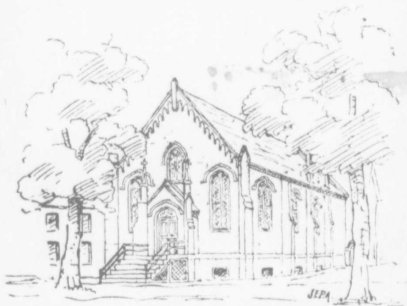
OLD CONGREGATIONAL CHURCH, BUILT 1858.
