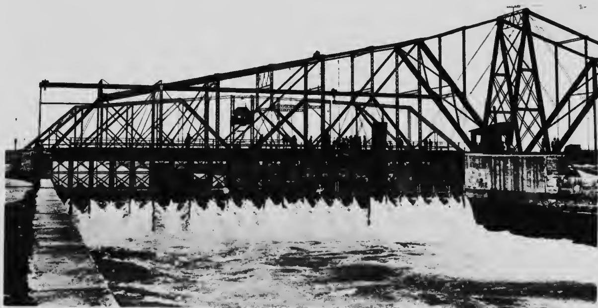
This illustration gives a view of the movable emergency dam built in 1895 for the Dominion Government at the Sault Ste Marie Canal for use in case of accident to the lock gates. The log frames can be lowered individually, and to any depth required, up to 30 feet (9.15 m).
