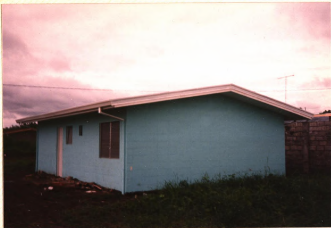
No. 69. Completed house, including exterior and interior finishing.
