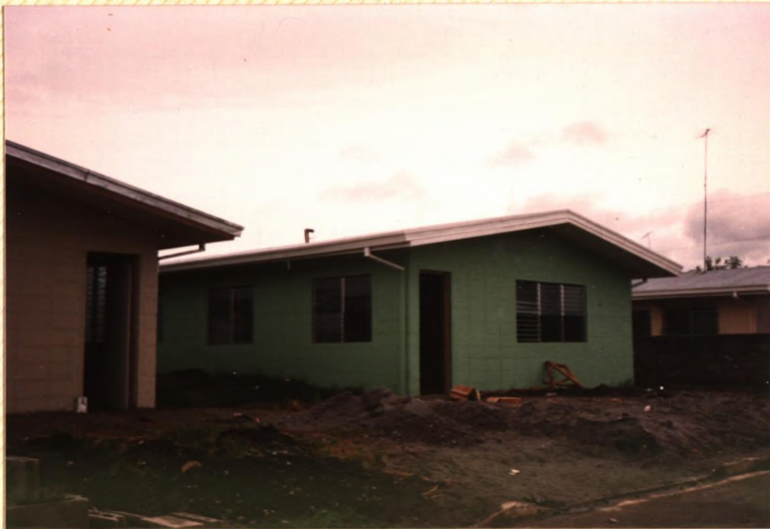
No. 68. House exterior complete, including glass jalousie windows.
