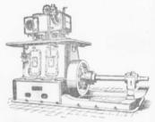
"We have used A Customer says: one of your Vartical High Speed Engines, English Type, forced lubrication, since 1907 The Engine runs at 425 revolutions per minue almost constantly night and day. It has given us every satisfaction and so far has cost us nothing for repairs."
