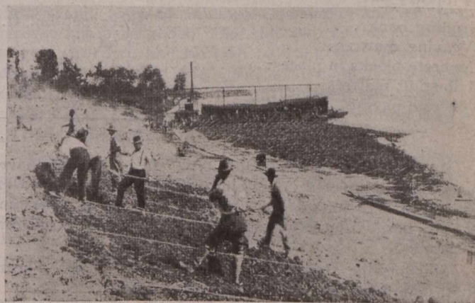
Fig. 4—Placing Concrete Blocks
