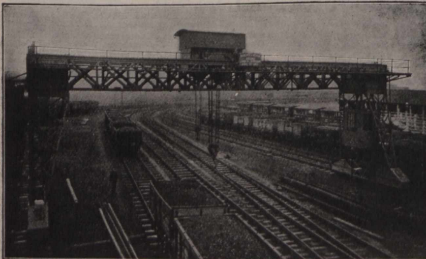
The G. & S. W. Rwy., Albert Harbor Goods Station, Greenock, N.B. "B. & W." 30 Tons Electric Travelling Goliath Crane, 70 Feet Span
