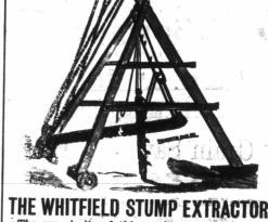
The superiority of this machine consists in the rapidity and ease in which it can take out the largest stumps; its great strength and durability; its easy operation by man or beast. It leaves no holes to fill up, or any stumps or stags in the ground
