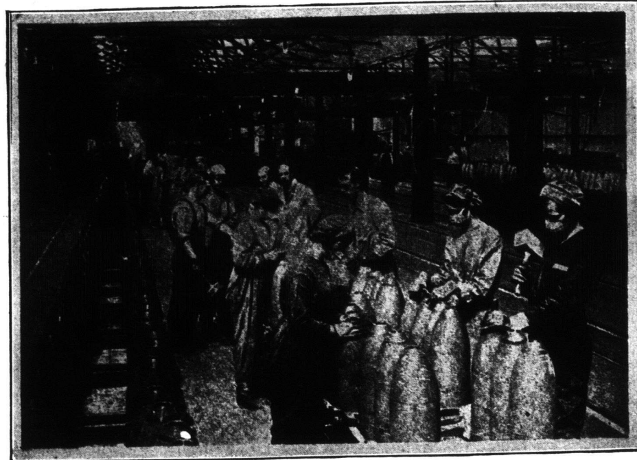
A trolley train doing duty between the various departments of a shell factory.
