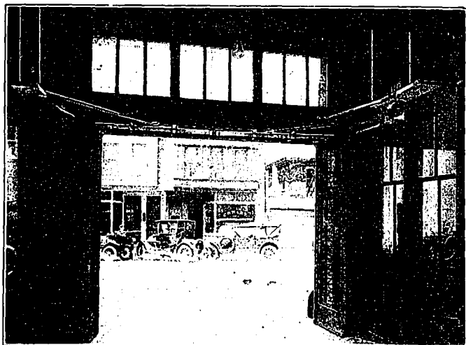
ELECTRICALLY OPERATED GARAGE DOOR.
