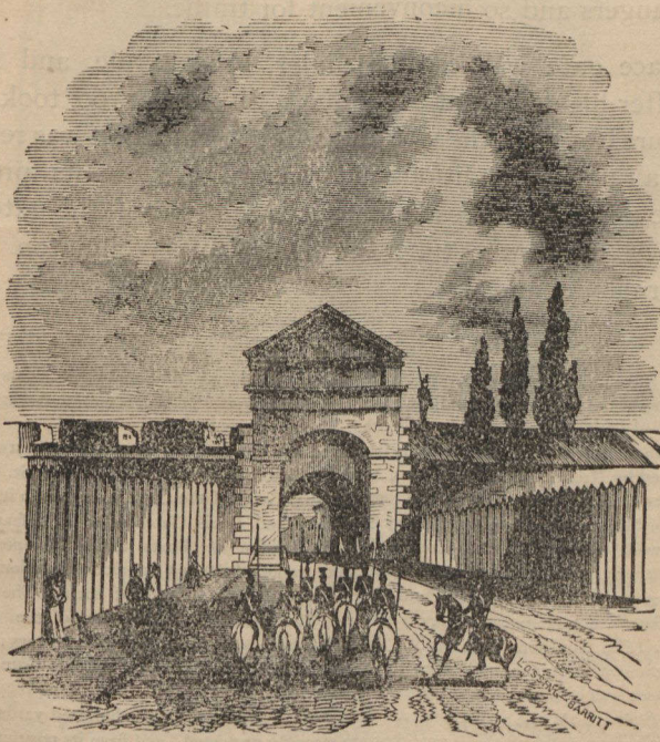
ST. LOUIS GATE, DEMOLISHED, AUGUST, 1871.
