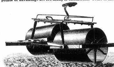
There is no axle shaft, no strain, and consequently no wear. It is easily oiled between the drums.
