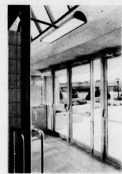
The variety of materials and textures is a pleasant relief from the omnipresent York brick and concrete.
