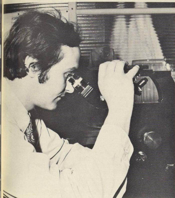
Dr. William Wallace of the National Aeronautical Establishment examines the microstructures of powder fabricated nickel-base superalloys. • Le Dr William Wallace, de l'Établissement aéronautique national, examine les microstructures de superalliages frittés à base de nickel.
