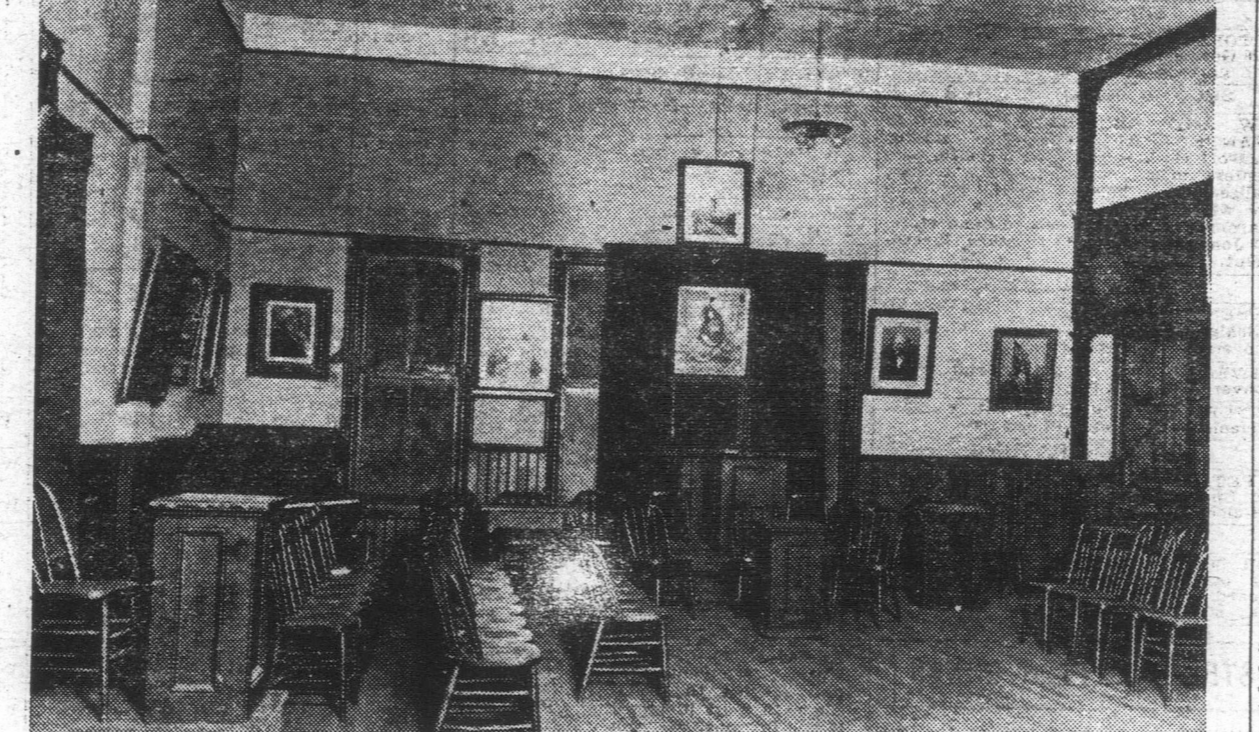
SIR WILLIAM WALLACE HALL. For the Last Time a Meeting of a Scottish Society Was Held in This Hall on Monday Evening. During the Night the Hall Was Damaged by a Fire Which Broke Out in the Roof of the Block. Caledonian Society Removed Its Effects From the Hall. Some of Its Pictures Are Invaluable.
