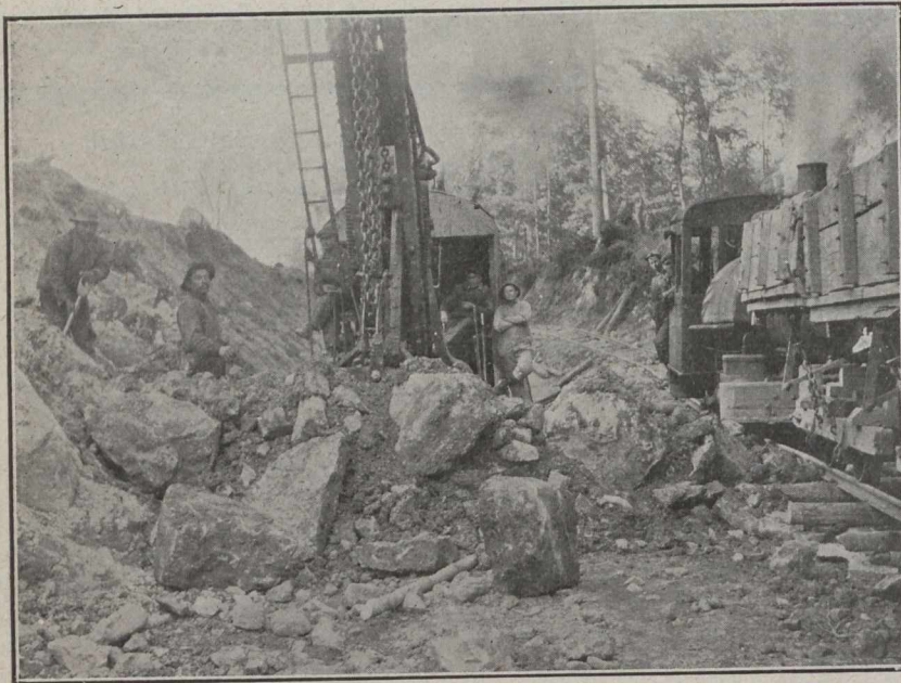
Flume Line Excavation, Providing Fill for Dam.
