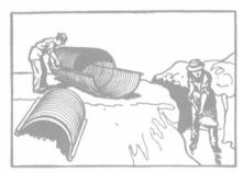
A few hours' work-no special skill needed—and an indestructible culvert is in place ready for use.
