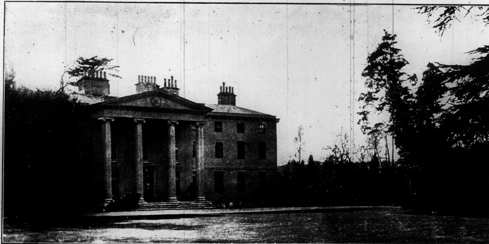
MAIN ENTRANCE, TEMPLE HOUSE, HURLEY LOCK.
