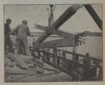
Fig. No. 2—Furness Withy Pier—Reinforced Concrete Brace Member
