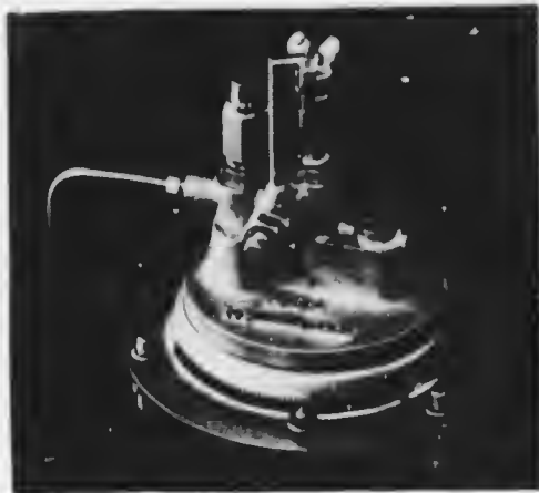
THE AGA FLASHING APPARATUS FOR RAILWAY SIGNALS
