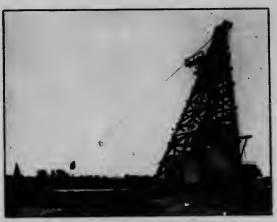
THE CABLEWAY EXCAVATOR HAS AN 800 FT. SPAN
