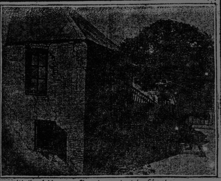
Walls of Mormon Church cracked by shocks
