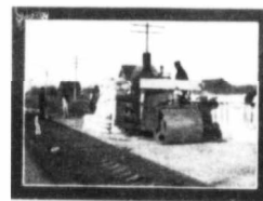
Testing Bridge for Heavy Traffic (St. Norbert)
