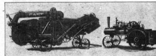
Case 40 H. P. Steam Tractor and 28x50 Thresher Fully Equipped A Medium Sized Big Capacity Rig
