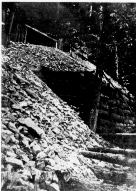
Ore Dump, No. 6 Tunnel Eva Mine.
