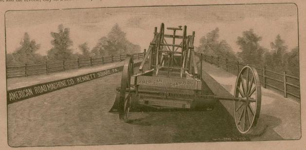
The above is The American Champion Reversible Road Machine—Rear View—showing the rear axle extended to the right hand, rear whee against the bank to prevent side-slipping in removing the earth from the ditch, shaving off hard, bony shoulders, etc.
