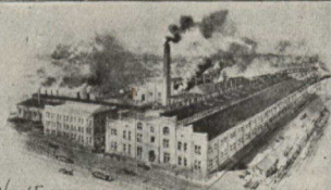
NEW FACTORY BUILT IN 1895 SINCE THEN THE FOLLOWING EXTENSIONS HAVE BEEN MADE MACHINE SHOP LENGTHENED 140 FT. NOW 440 x 120 BOILER SHOP 100 FT. NOW 220 x 80 WITH CORRESPONDING INCREASE MOULDING SHOP 100 FT. NOW 180 x 80 IN EQUIPMENT BLACKSMITH SHOP 40 FT. NOW 100 x 40
