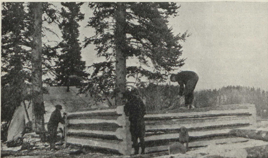
Fire Ranger's Cabin in Course of Construction.
