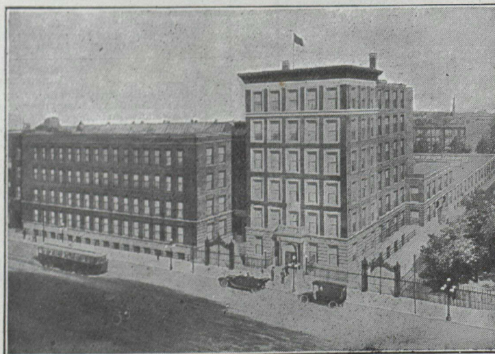
FIRE PROOF BUILDINGS
