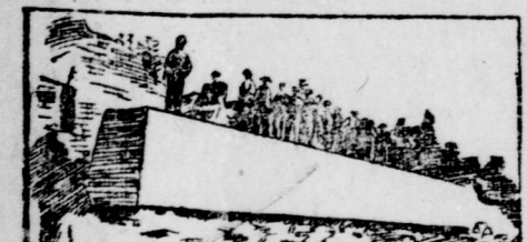
BLOCK OF GRANITE FOR ONE OF THE COLUMNS—WEIGHT 310 TONS; LENGTH, 67 FEET; HEIGHT, 84 FEET; WIDTH, 7 FEET.
