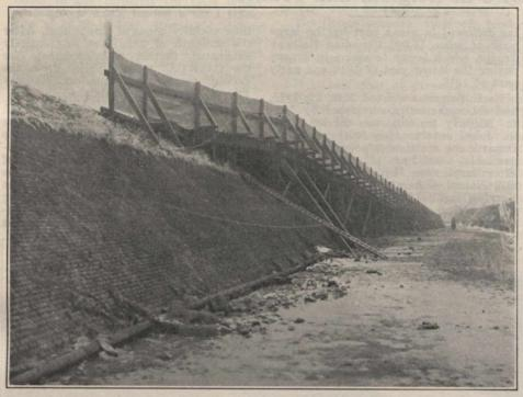
Side view of Timber Ramp, from towpath, to dry bottom of Canal du Nord, to permit it being used as a highway for artillery and team transport. Built by Canadian Overseas Railway Construction Corps, Nov., 1917. The embankment was approximately 40 ft. high.
