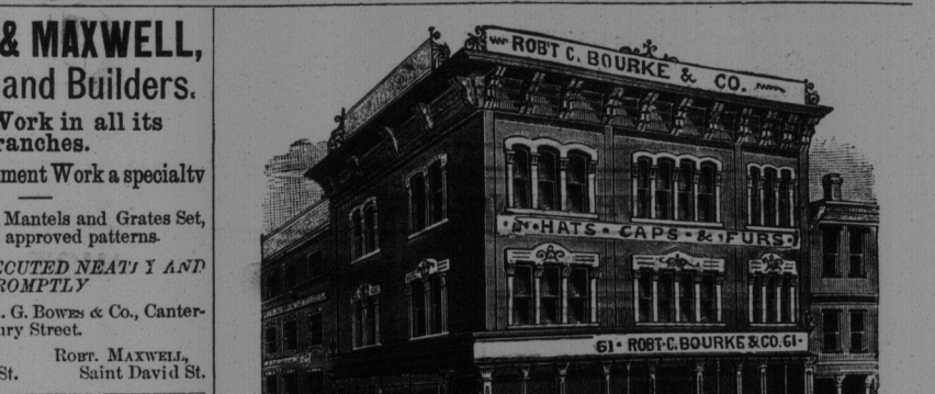
ROBT. C. BOURKE & CO. BOILERS, RANGES, MANTELS AND GRATES SET.
