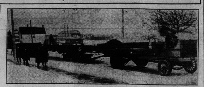
Forty tons of steel for the St. Clair avenue bridge, being handled by an auto truck up Shaw street grade near Davenport Hill. The sections are nearly 100 feet long, and the truck had four tons of steel aboard to give it traction. The total weight, including the sleighs, was nearly 60 tons.
