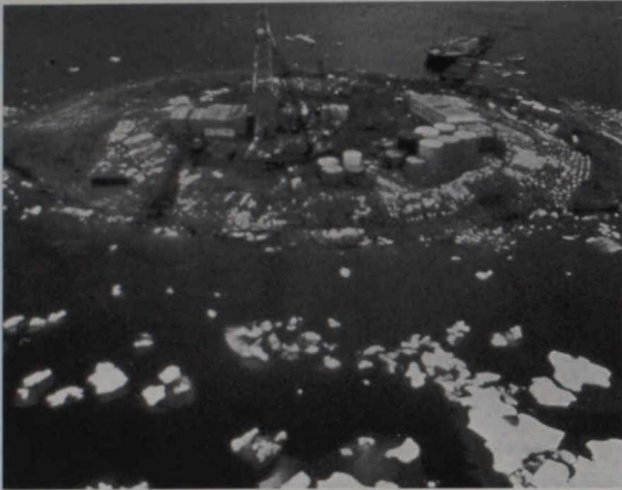
Esso's artificial island at Issungnak.
