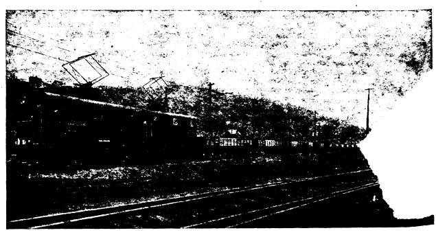
135 Ton Westinghouse Single-Phase Freight Locomotive, Hauling Train of Fifty 50 Ton Steel Frame Gondola Cars.
