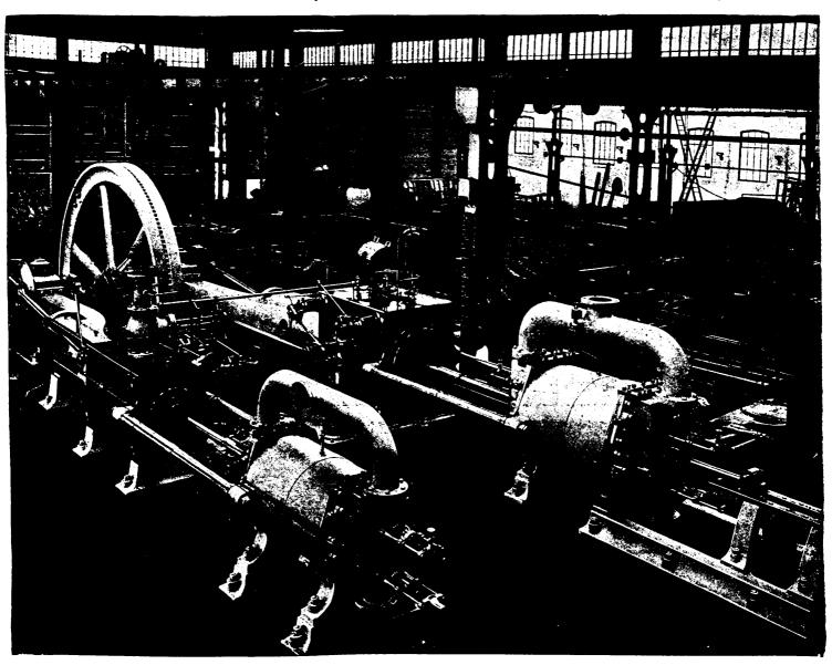
WALKER BROTHERS HAVE RE-MODELLED OVER 100 AIR COMPRESSORS ORIGINALLY CONSTRUCTED BY OTHER MAKERS.
