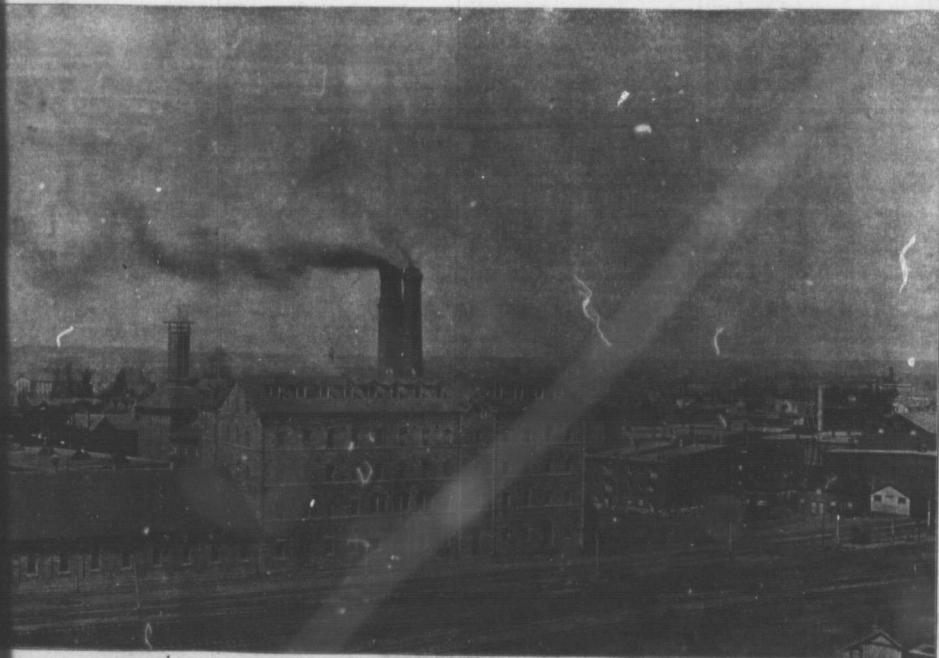
GENERAL VIEW OF THE PREMISES FROM WATER FRONT
