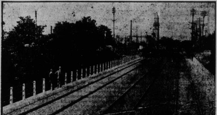
THE double tracking of the North Toronto Sub-division of the Canadian Pacific Railway between Leaside and North Toronto is now nearing completion, and involves the replacement of bridges (known as 0.3 and 1.3) which heretofore had been trestles constructed of steel. Owing to the high price of steel and the difficulty of procuring it since the war began it was found that reinforced concrete competed successfully against steel.
