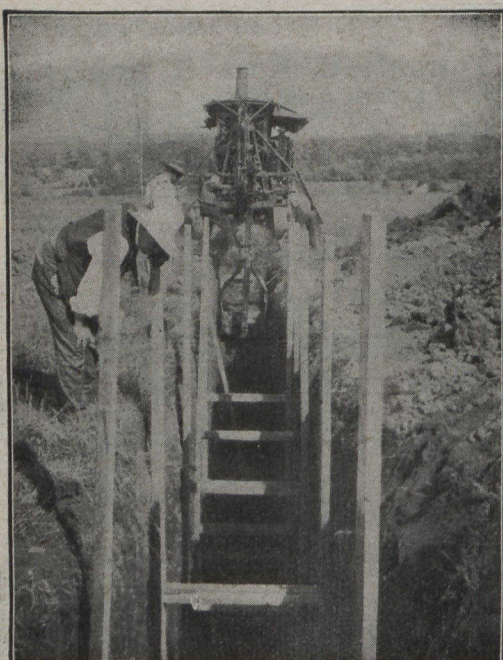
A Keystone Excavator, Model 4, at ditching—96 feet long, 14' 6" deep and 40" wide in one day. No hand trimming necessary.
