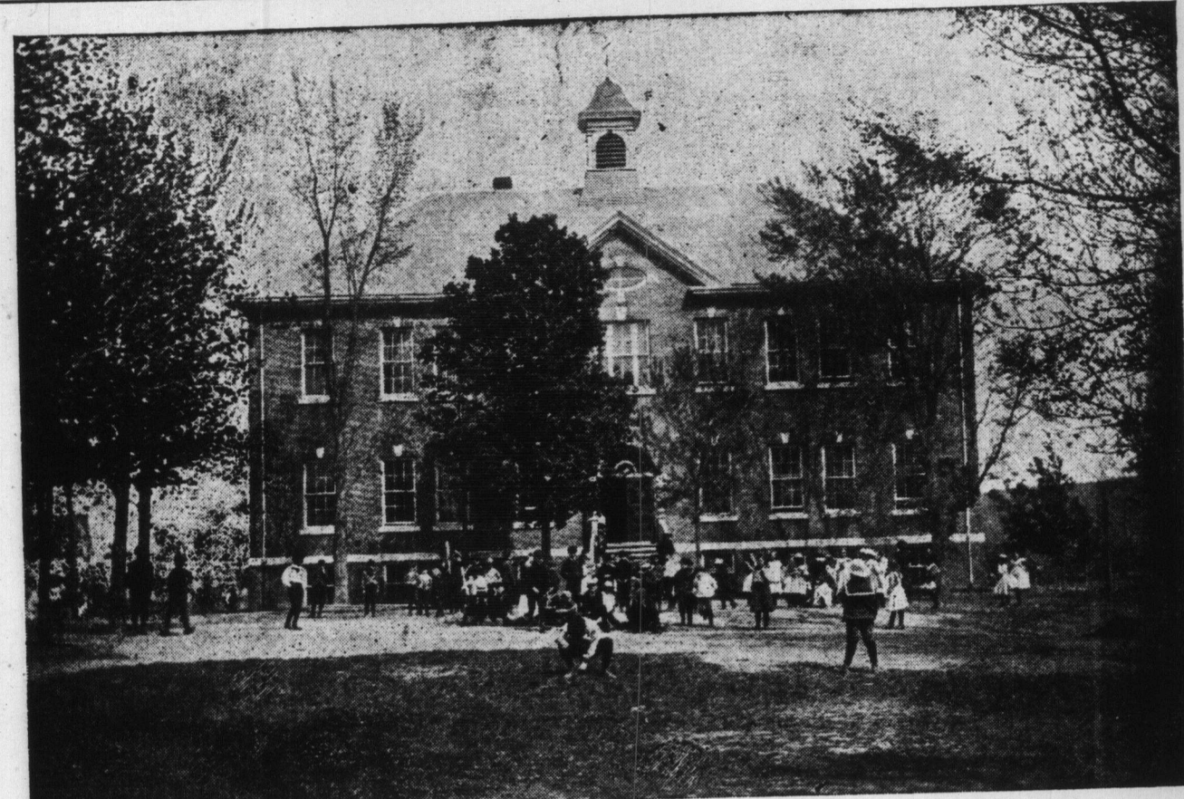
THE BRIDGETOWN SCHOOL BUILDING
