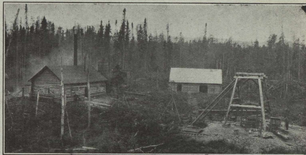
The Wasapika Power House and Head Frame.
